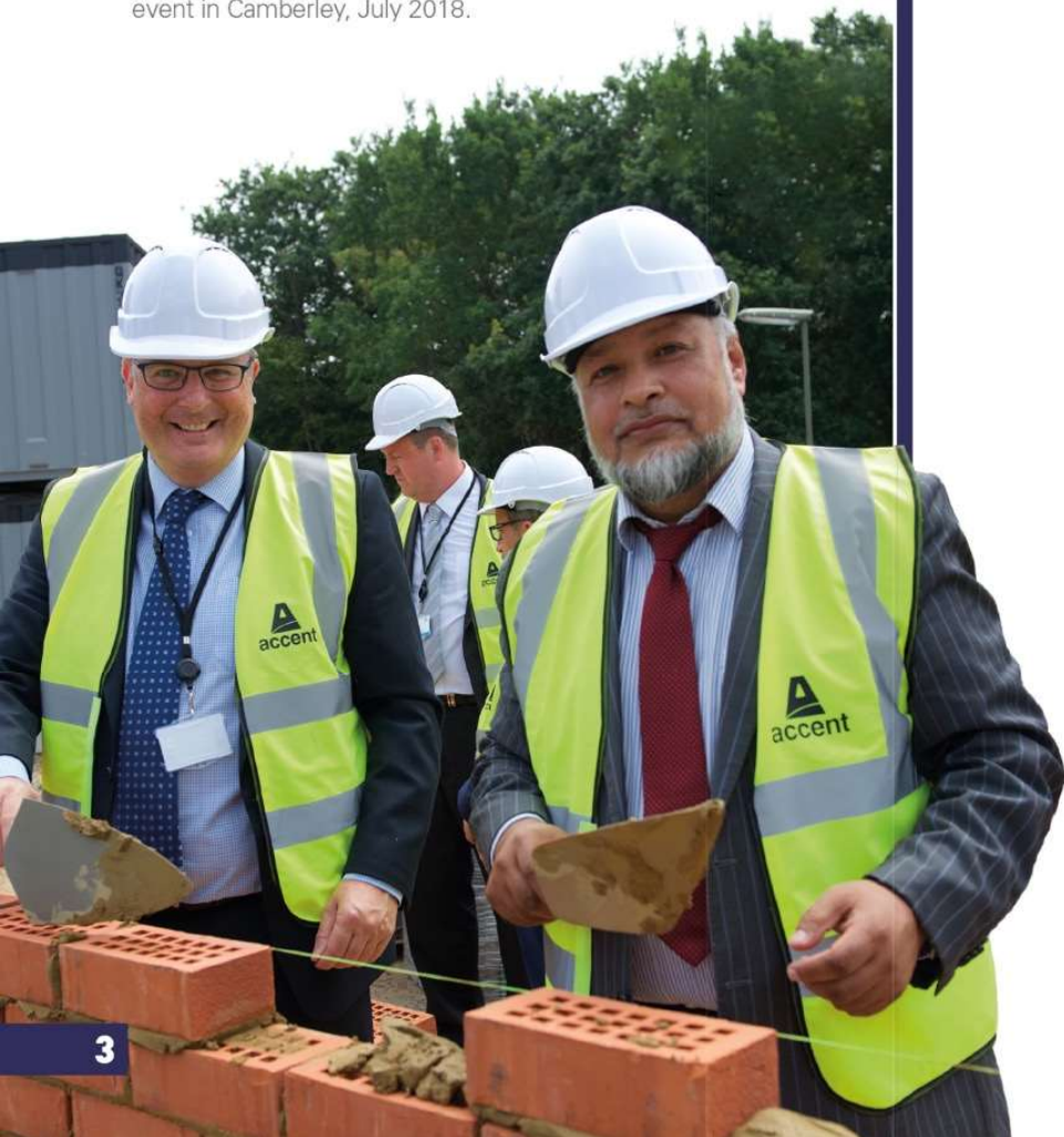
Robert Mills, Regional Housing Director (left) and Jamir Ali, Project Manager (right) during a start-on-site event in Camberley, July 2018.
